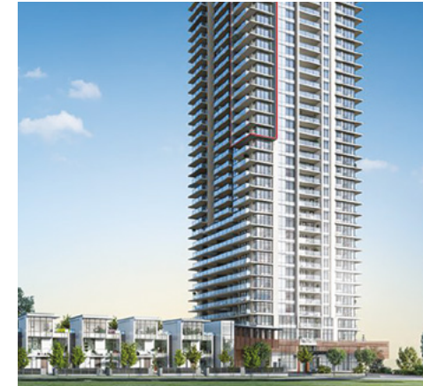
FULTON Burnaby, BC Frigate ERV 100 DS Quantity: 98 Frigate ERV 120 S Quantity: 208
